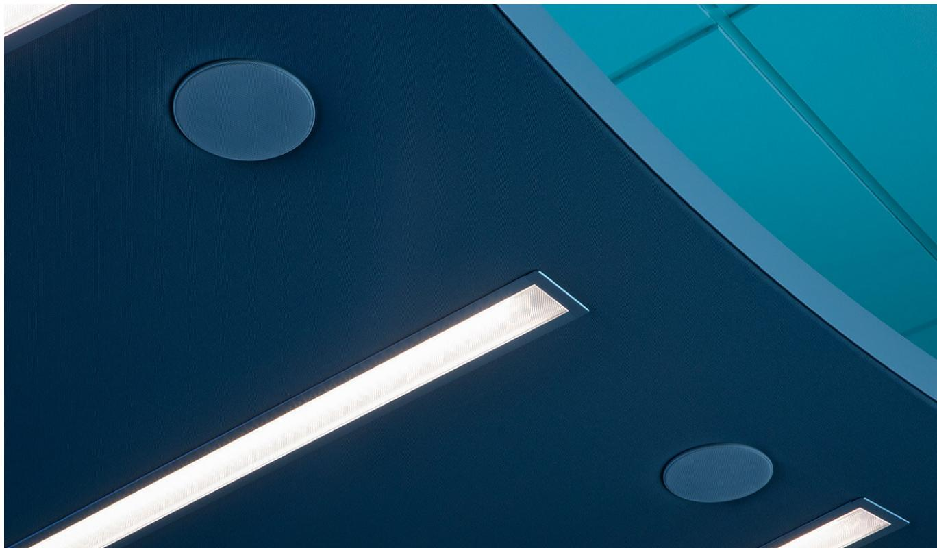
Exciting attributes of the acoustic ceiling sail (here in the control center of Heidelberg Materials in Ennigerloh): The integrated audio system of the Opal X11® can be controlled via the JST user interface myGUI® as well as optionally via Bluetooth. The link with myGUI® also triggers the AlarmLight in the case of an event – either by lighting up or flashing, depending on the presetting. Malfunctions are thus perceived both auditorily and visually.
