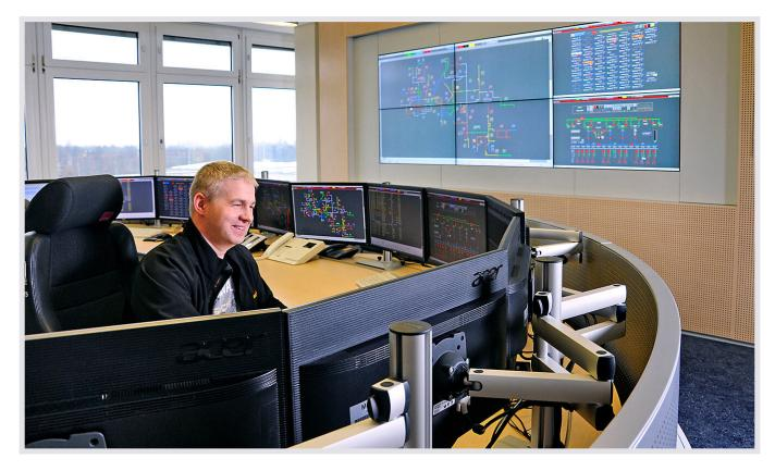
JST <u>DisplayWall</u>: A large display wall visualises the most important events for the operator team in the technical control center of the "Competence Center Surface".
