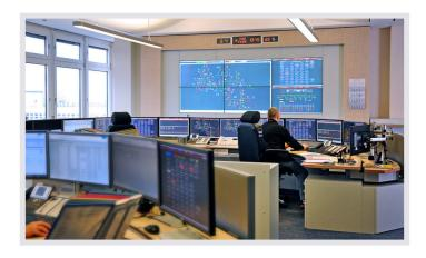
JST-MultiConsoling®: The heart of the technology is MultiConsoling®, with which all computers from the control center could be installed in a remote technology room. Advantage: less heat, less noise. In addition, the computers are – depending on access authorisation – arbitrarily connected by the operators to the <a href="large display wall">large display wall</a> and the monitors at the workplace and operated in real time.
