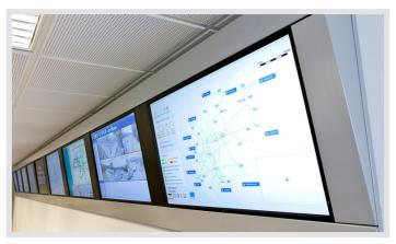
**Optimal space planning** – the <u>large-screen displays</u> are positioned high enough so that the operator can follow what is happening on the large display wall across the second screen level at the workstation.
