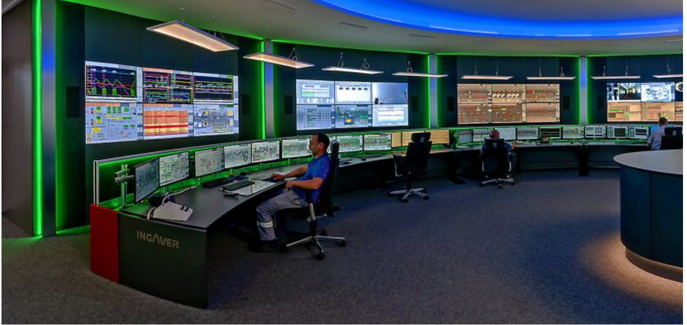
Virtual 360° tour through the control room.
