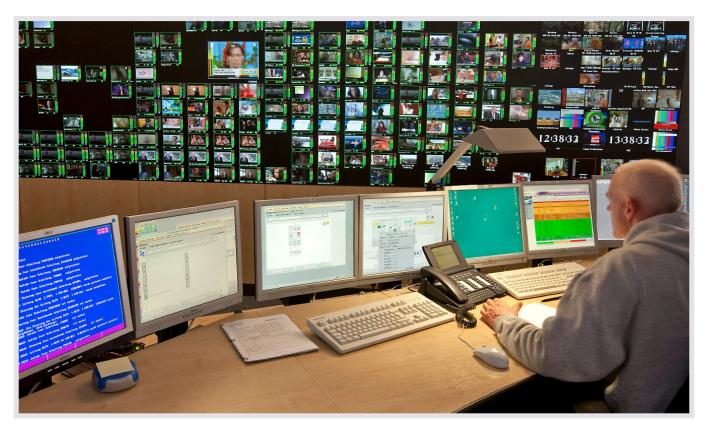
The integration of a video rear projection screen with over 250 TV images and the new proactive display wall with large variably interconnected LC displays was another challenge for JST.
