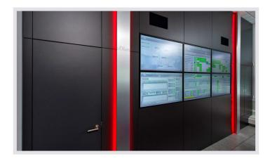
JST large screen wall: Directly next to the displays on the <u>large screen wall</u> is a door that provides access to the newly created room-in-room – a special JST solution that keeps heat and noise away from the control room.
